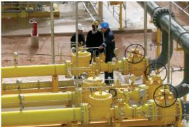
Today's natural gas industry has a growing demand for operational excellence. Pilot-operated gas regulators must provide reliable performance in applications ranging from gas distribution systems, to gas-fired power plants and processing facilities. The regulators are also employed in commercial and industrial gas service.
