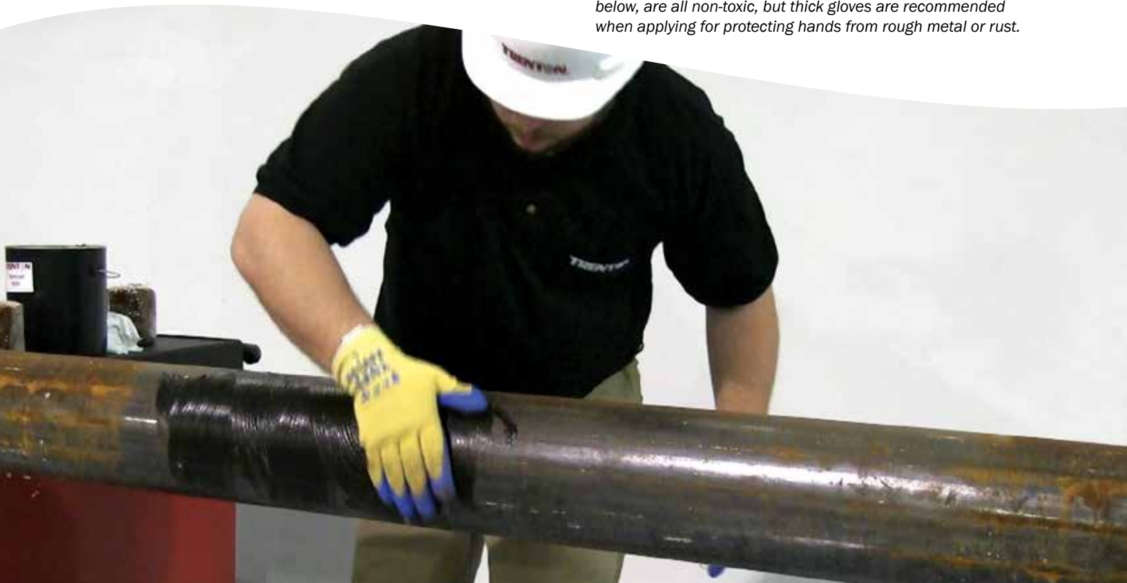
Here Trenton's Wax-Tape® #2 wrap is being applied over the Wax-Tape® primer (white). Notice that the Wax-Tape primer can be applied to the pipe after only minimal surface preparation.
