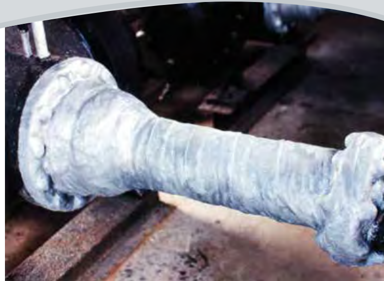
A sweating meter run pipe protected with Wax-Tape® #2A wrap demonstrates the wraps's ability to protect in wet conditions.
