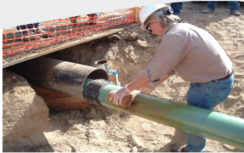
Wax-Tape HT-3000 wrap does not require sandblasting. Here the wrap is being applied to moderate-temperature pipe, but it can also be applied to hot in-service lines by using insulated gloves.
