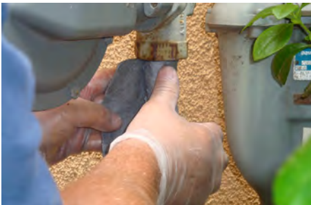
7. Starting at the bottom of the riser, firmly press the Wax-Tape® wrap around the pipe with the seam facing toward the back of the pipe. When using additional pads, use a minimum of 1" overlap.
