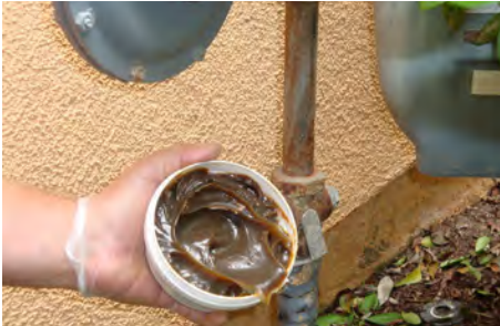
4. Hand apply the primer. Firmly rub and press the primer onto the surface to displace the moisture and ensure that the primer is adhering to the metal surface.
