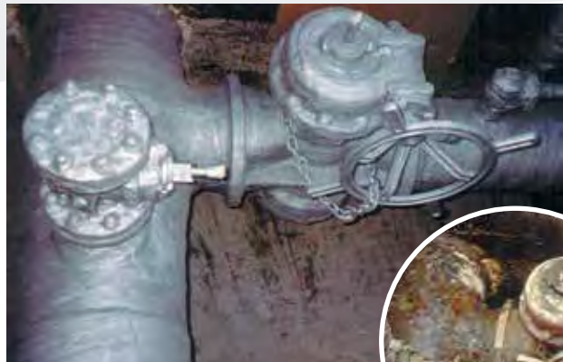
Trenton Wax-Tape® brand anticorrosion wraps, such as Wax-Tape® #2 self-firming anticorrosion wrap, excel in limited-access situations, such as vaults, where surface preparation is difficult.
