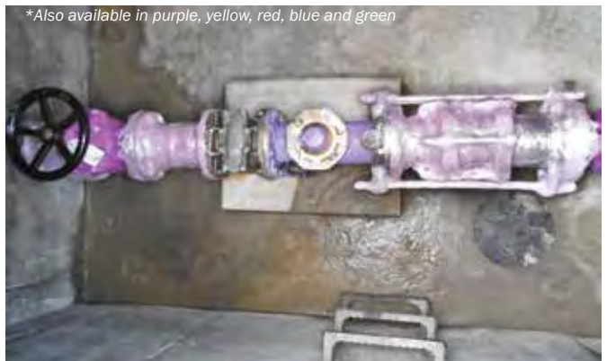
Wax-Tape® #2 anticorrosion wrap is available in many colors. This pipe is wrapped in purple tape, often used in the water industry. Wax-Tape #2 wrap meets AWWA C217 2016 standards.
