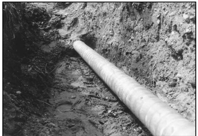
Section of 16" pipe reconditioned using #1 Wax-Tape and Glas-Wrap.
