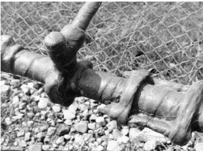
#1 Wax-Tape applied to coupling, street tee and leak clamp.
